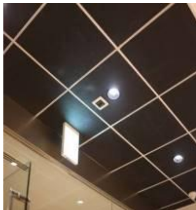
Picture 22 : Robot Eye sensor located at the main entrance of the Exhibition Center
