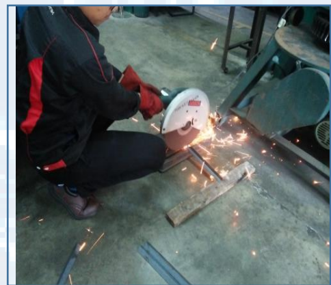
Figure 5(b): The mild steel plate has been cut by using power saw.
